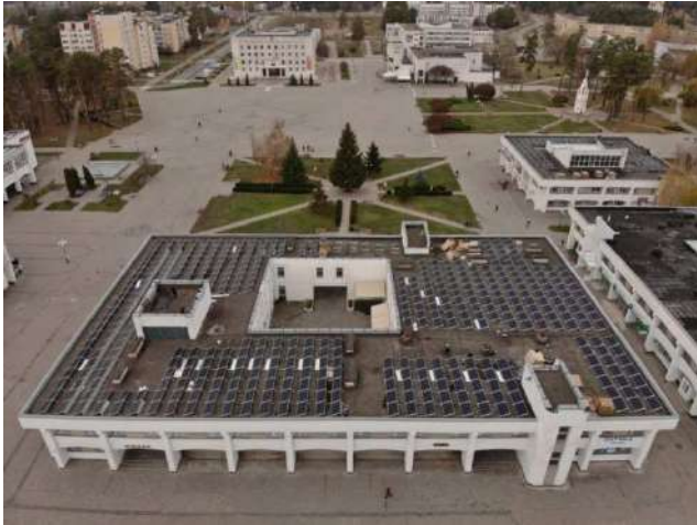
View on one of the solar power-plants of Solar Town municipal energy coop
